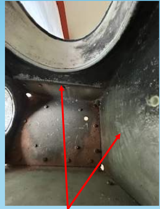
Membrane marks on airbox walls
